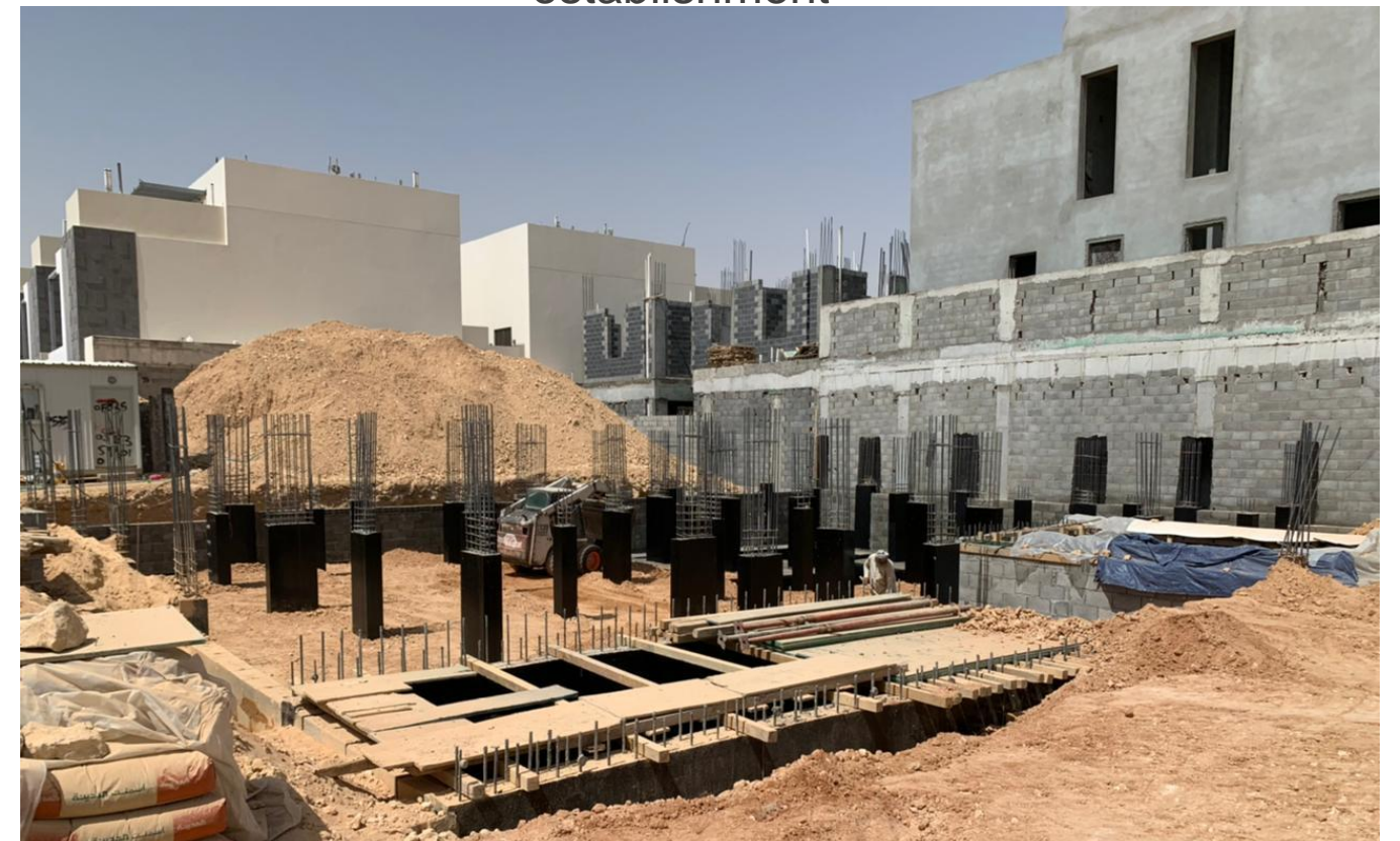
Determine the filling layers on the pad foundation, as well to the columns and start filling work
