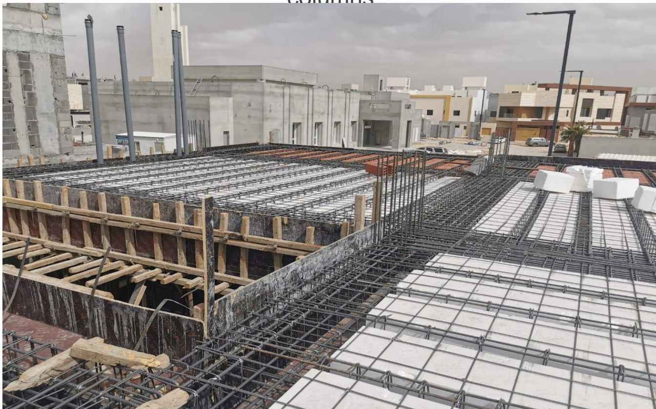
Carpentry, blacksmithing and pour concrete to the ground floor's roof
