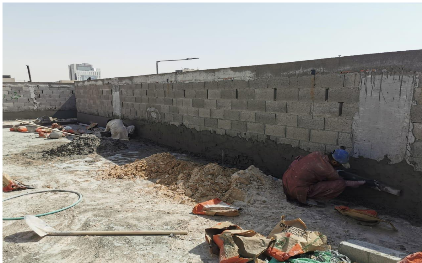
Plaster works with wall isolation
